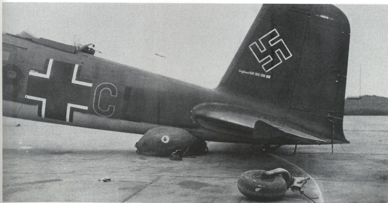
Below: After twenty missions flown over the North Sea, the Bay of Biscay and the Atlantic Ocean, this Fw 200 C shows light damage after returning from a long-range mission. After lifting the rear part of the fuselage, the aircraft was brought to the Feldwerft to be repaired quickly since only minor damage had been reported.
